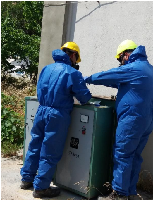
Figure 16: Sampling of PCB containing devices by specialized personnel, at MJT airport
